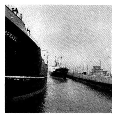
four 10,000-ton vessels at a time, giving it a capacity four times that of the old lock. Because of the elimination of delays, which formerly lasted as long as 18 hours at times of heavy traffic, substantial savings are already being achieved by ships using the port.
